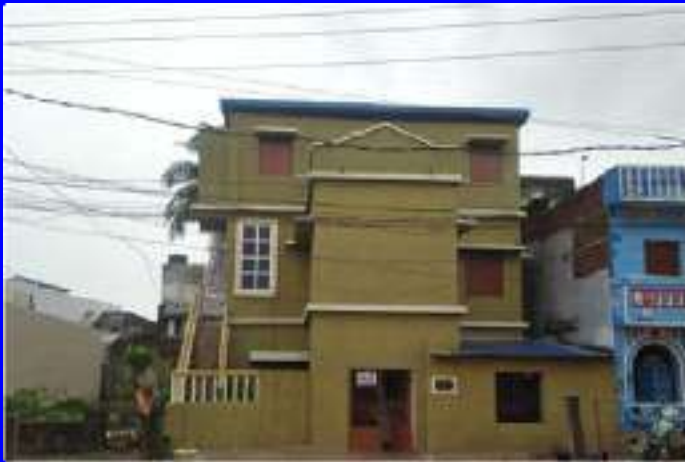
SWAD Building at Berhampur
